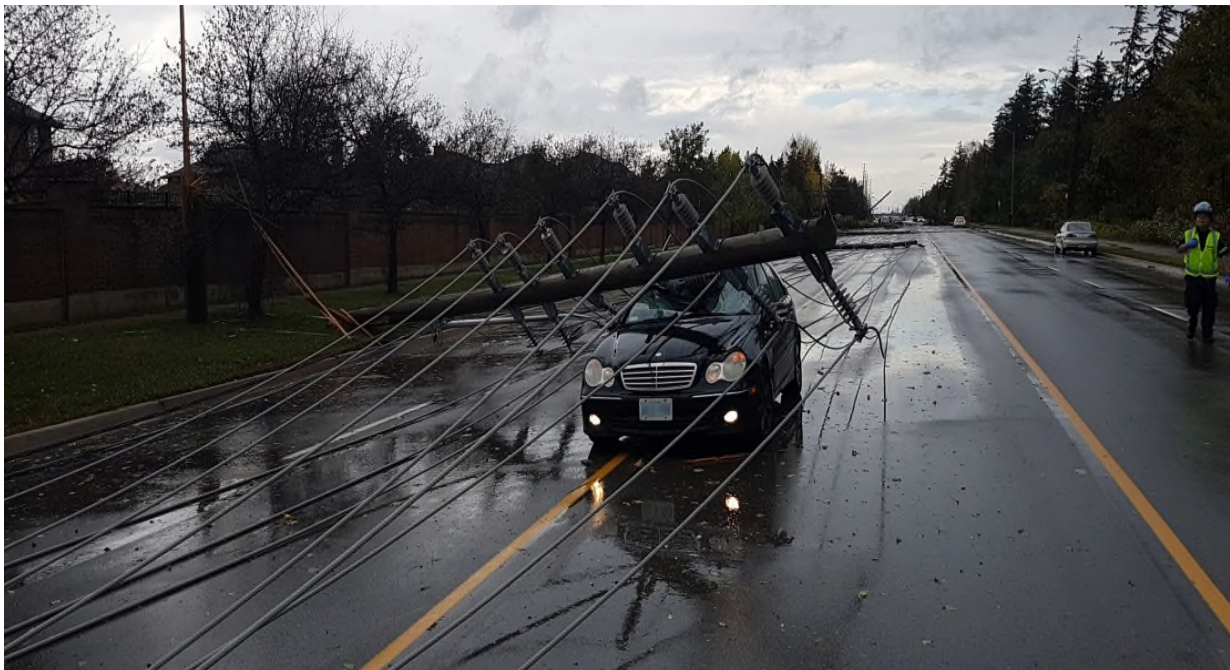
Figure 1: Failure of Wood Pole on October 15, 2017
